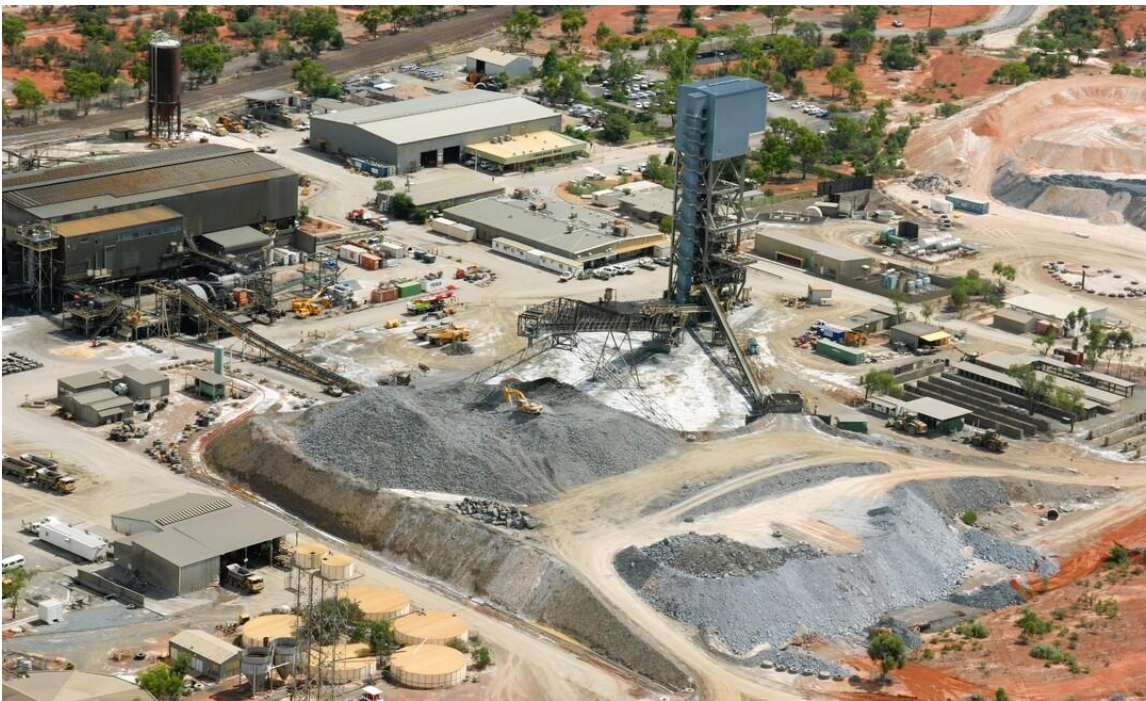
Endeavor mine surface infrastructure
